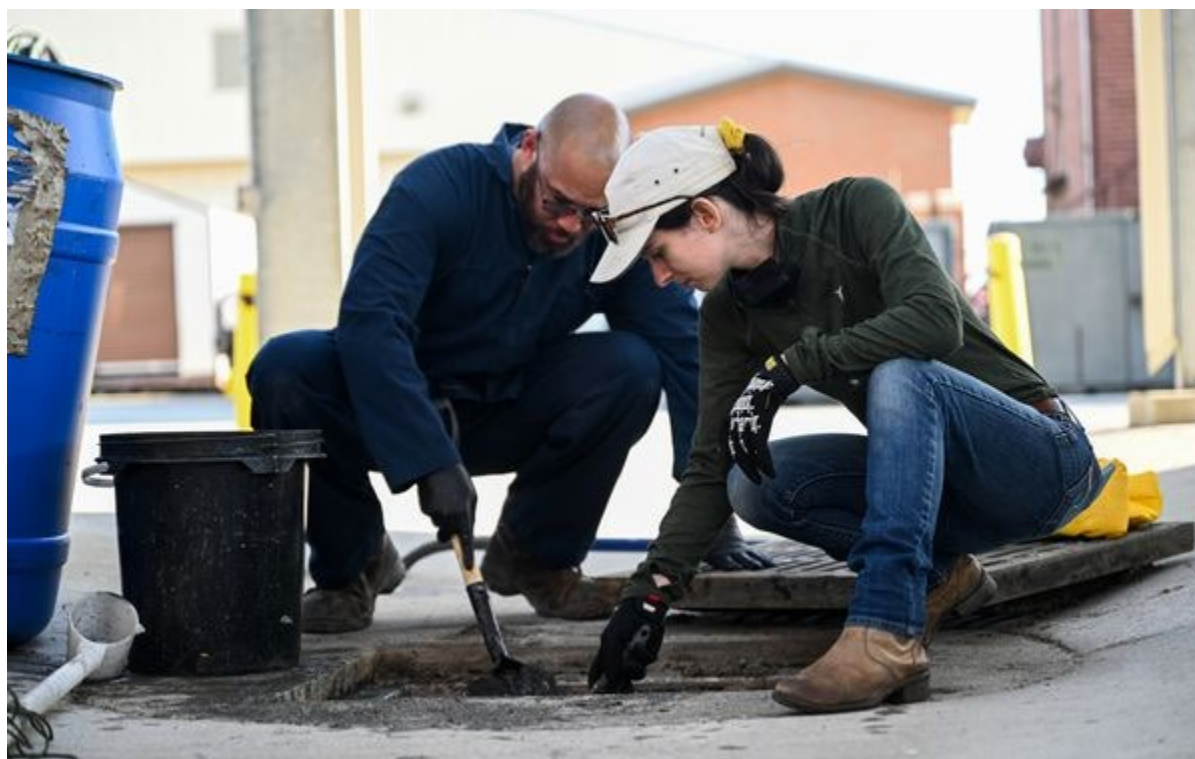
Figure 4-4. JBLE–Langley Staff Replacing a Safe Drain Water Filter
