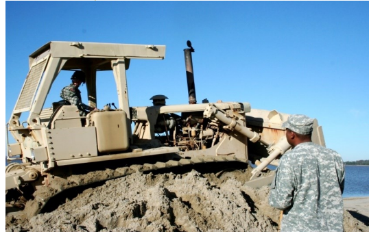
Duck pond excavation training at Fort Eustis, VA Training Area 18.
