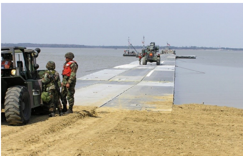
Successful excavation, pier stab and logistics over the shore training exercise.
