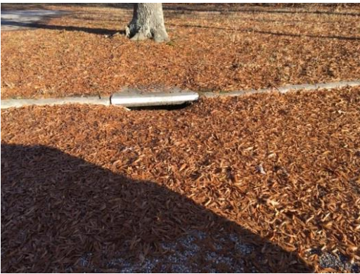
Photo 1205-3. Leaf litter debris entering storm drain (1)
