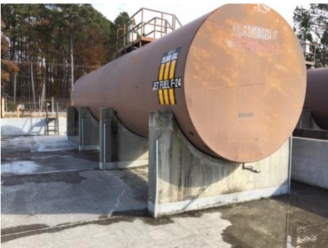
Photo 2451-3. Field-constructed AST #1
