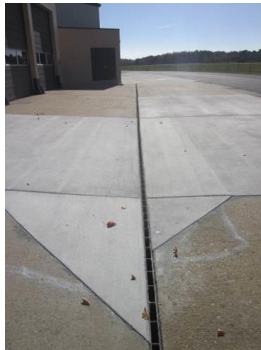
Photo 2401-3. Outdoor trench drain
