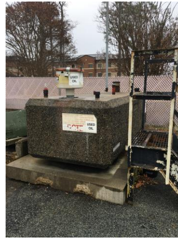
Photo 2702-4. Used oil tank
