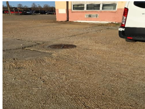
Photo 1406-3. Sand and sediment entering storm drain
