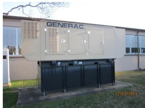
Photo 1407-2. EDG and associated AST
