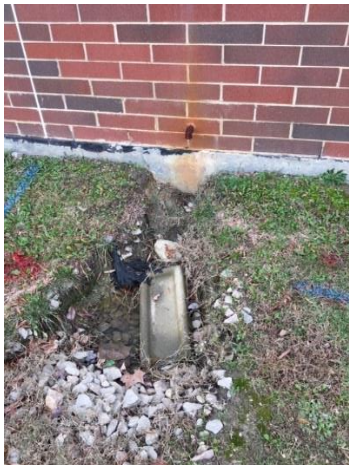
Photo 703-3. Erosion/wash out
