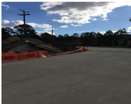
Photo 410-1. Construction silt fence
