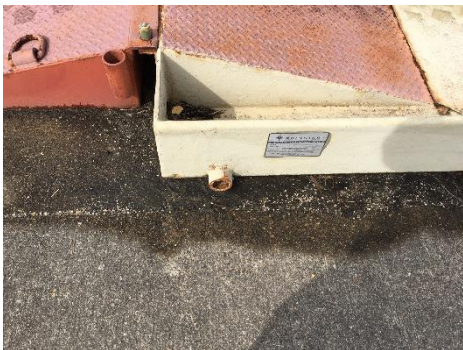
Photo 2449-5. Fuel truck secondary containment plug missing
