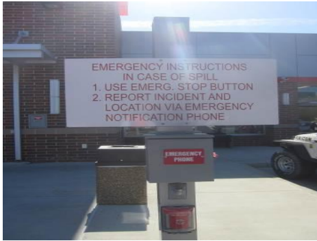
Photo 704-4. Emergency shut off for pumps
