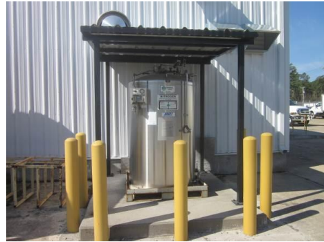
Photo 3528-2. Nitrogen tank (covered)
