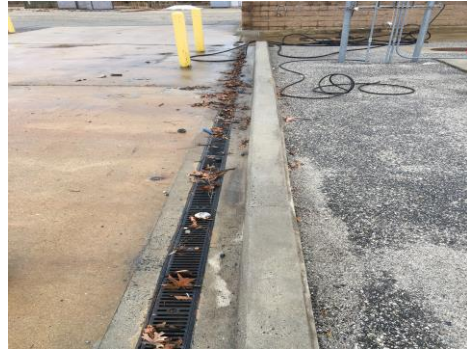
Photo 2705-2. Mud rack drain restricted
