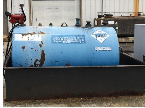
Photo 1423-4. Fuel tank in secondary containment
