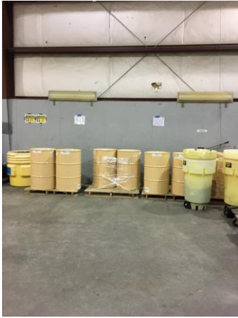
Photo 845-1. Drums of oil not stored on secondary containment
