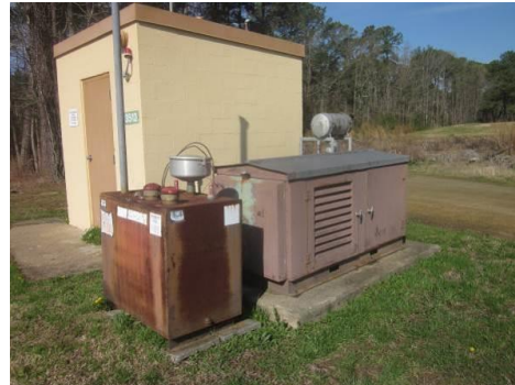
Photo 3512-1. Diesel AST for generator (3512-1)
