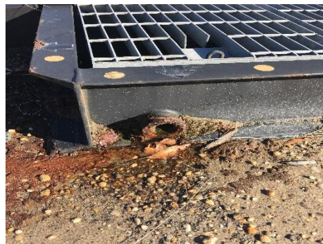
Photo 2705-4. Secondary containment drain plug missing
