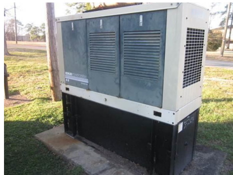
Photo 2713-2. EDG for lift station
