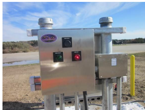
Photo 2449-2. Wash rack control panel
