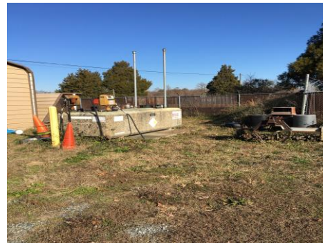
Photo 1428-4. Diesel/gasoline dual-chambered AST
