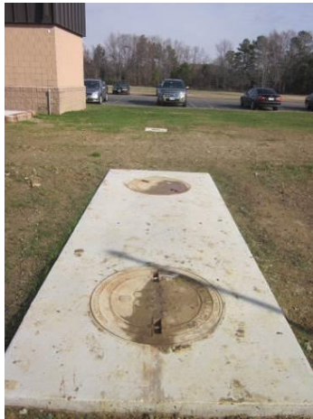
Photo 2414-3. Stormwater diversion valve pit
