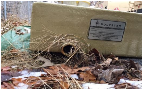
Photo 1035-3. Secondary containment drain plug missing
