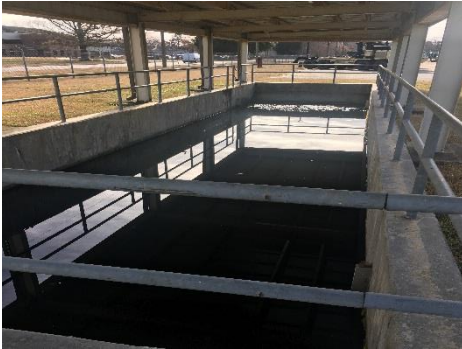
Photo 2508-2. Holding Tank for OWS
