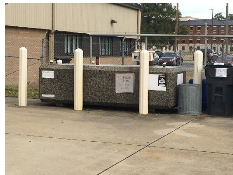
Photo 2505-3. Used oil AST (Tank 2505-1)
