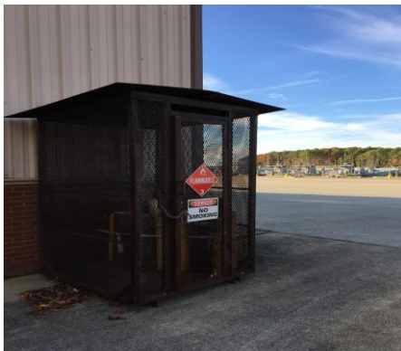
Photo 455-3. Compressed gas storage (2)
