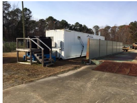
Photo 1411-10. Outdoor wash rack with recycling system
