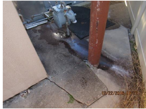
Photo 2407-2. Condensate discharge
