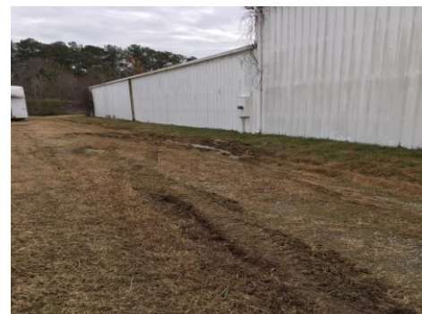
Photo 3523-5. Ruts caused by equipment
