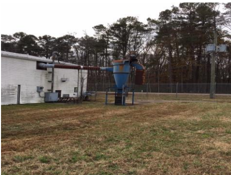
Photo 3509-2. Saw dust collection unit
