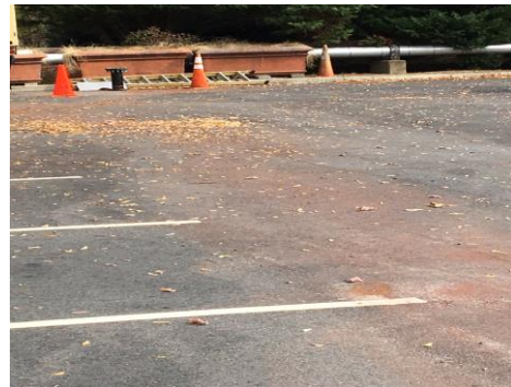
Photo 587-4. Sediment build up
