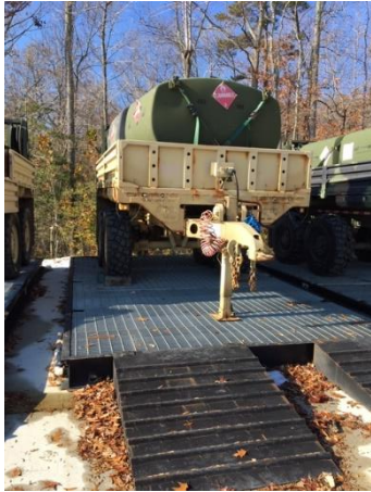
Photo 886-1. Mobile fuel tank secondary containment
