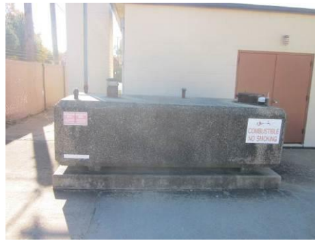
Photo 816-1. Heating oil AST
