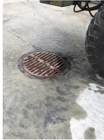
Photo 888-1. Storm water inlet contains sediment
