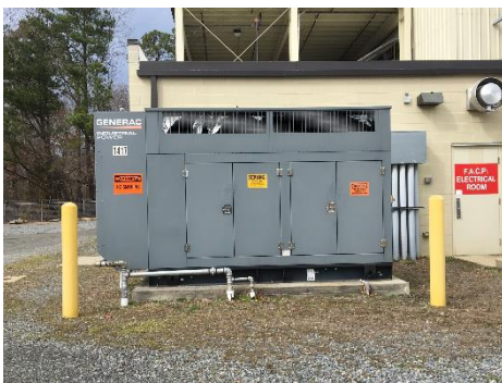
Photo 1417-1. Paint booth emergency generator
