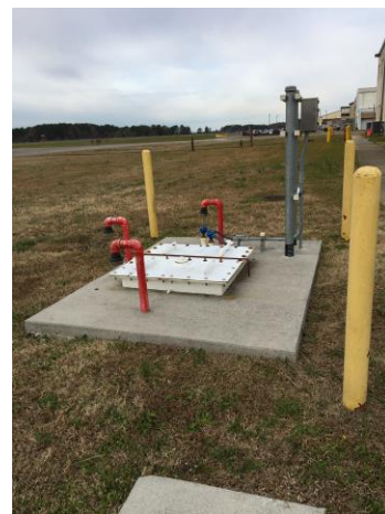
Photo 2413-6. Oil/water separator
