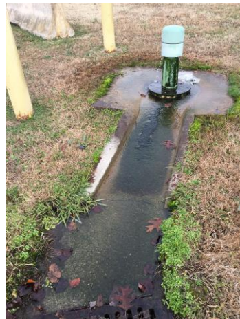
Photo 2450-1. Potable water auto flusher
