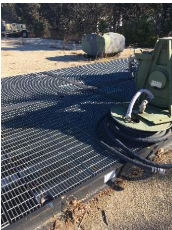
Photo 2705-3. Secondary containment
