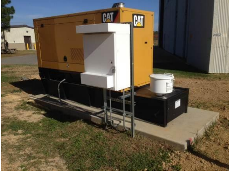
Photo 2401-1. EDG and associated AST
