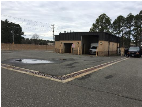
Photo 2742-1. Outdoor trench drain
