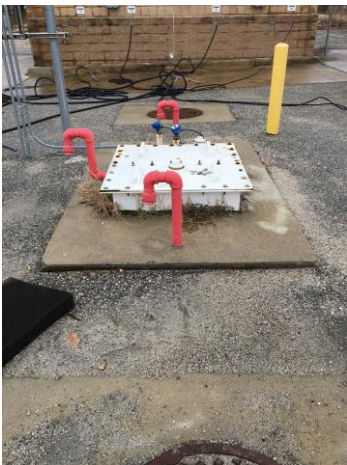
Photo 2705-2. Oil/water separator
