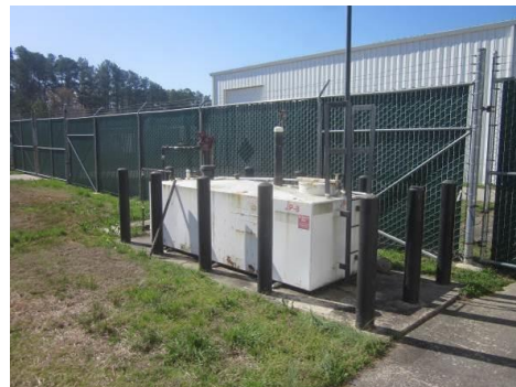
Photo 3517-2. Jet A AST for engine testing (3517-1)
