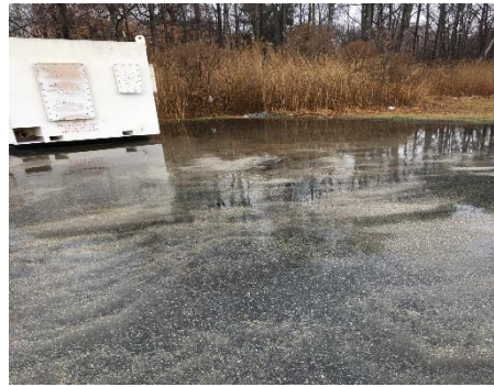
Photo 211-2. Sediment build up
