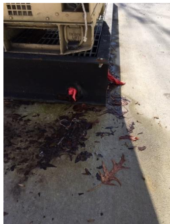
Photo 888-2. Equipment storage secondary containment missing drain plugs
