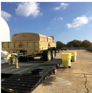
Photo 836-5. Secondary containment with storm water
