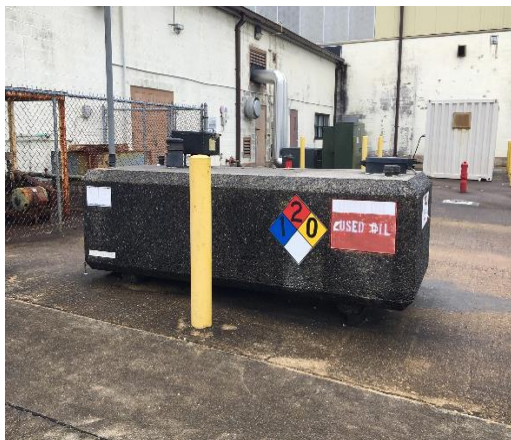
Photo 836-3. Used oil tank
