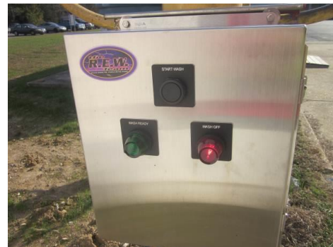
Photo 2414-6. Wash rack control panel
