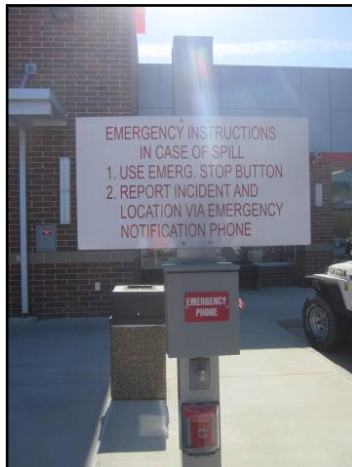
Photo 704-3. Emergency Shut Off for Pumps
