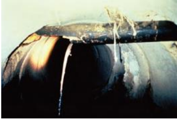
Sewer Pipe Leaking into a Storm Pipe
