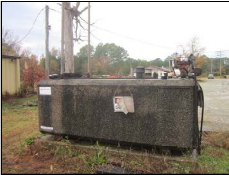
Photo 3534-1. Diesel and Gasoline AST (3534-1)
