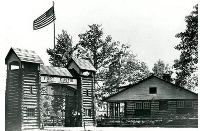
Photo: Historic photograph of the Fort Eustis gates.
