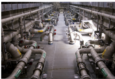
Filter gallery pipes at our Lee Hall Water Treatment Plant.
