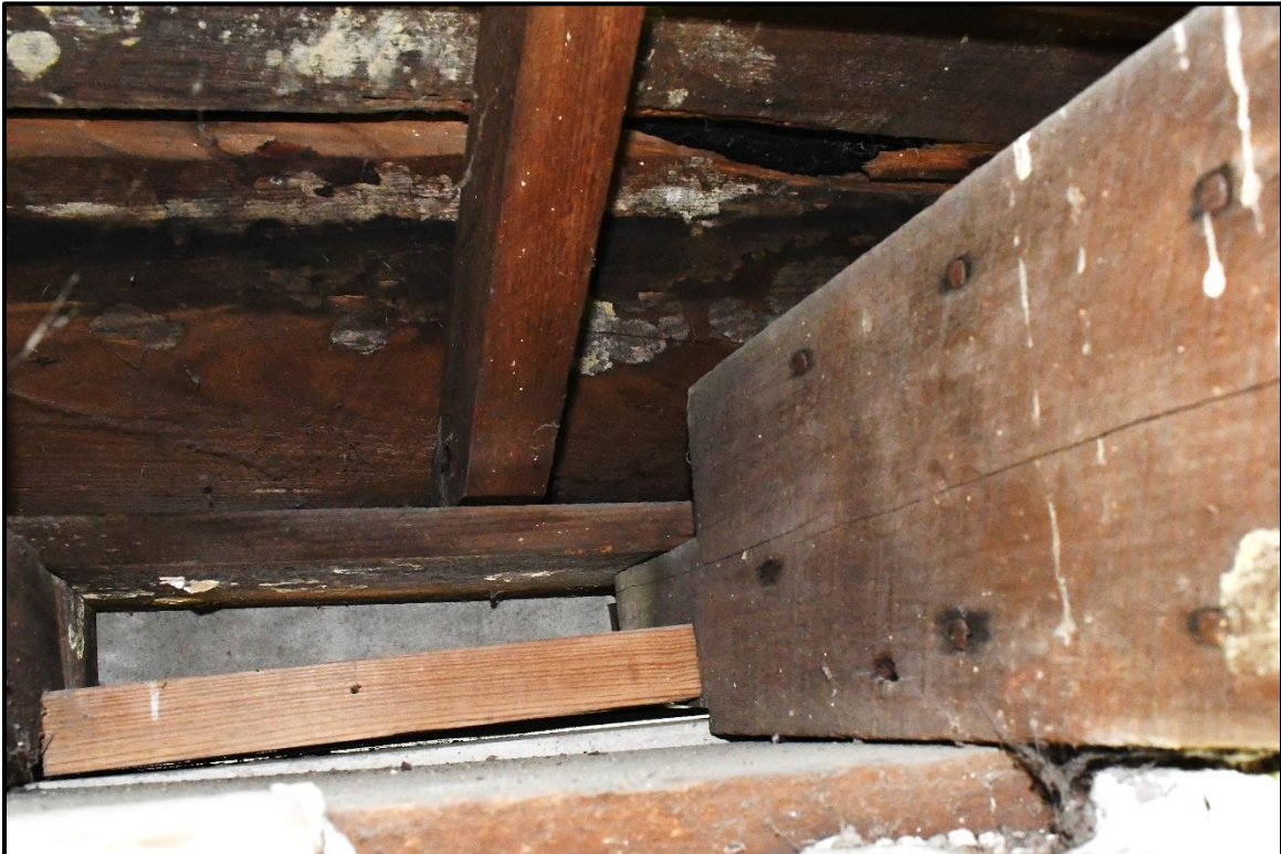
Photo 24: Main roof rafter and attic floor joist bearing condition located at the north wall of the home.
