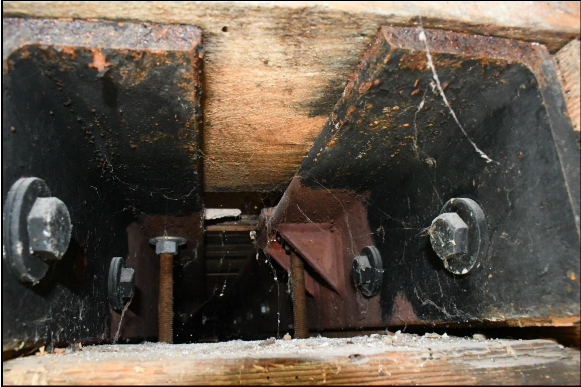
Photo 29: Steel angles installed adjacent to the second floor joists and hung from the steel beam located above the main roof attic joists.
