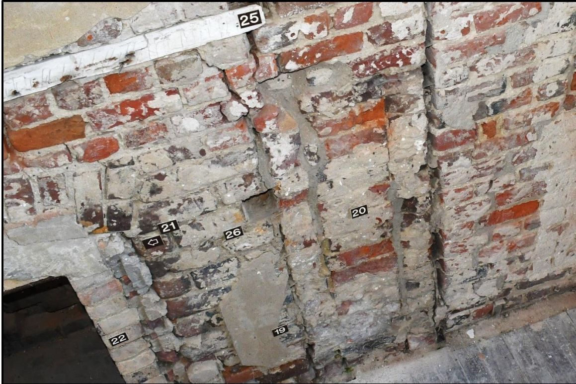
Photo 19: Typical condition of the masonry located on the interior surface of the west gable end wall. Note the joints between the varying wall segments.
