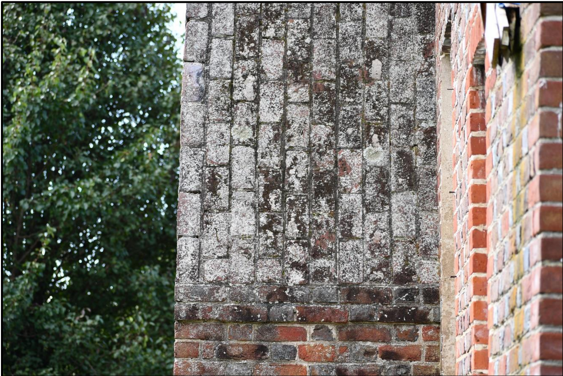
Photo 16: Significant presence of organic growth located at the sloped surface of the east elevation chimney.
