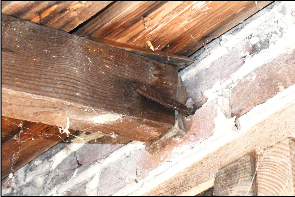
Photo 25: Upper connection of the rear shed roof rafter. Note the corrosion on the original framing hardware.
