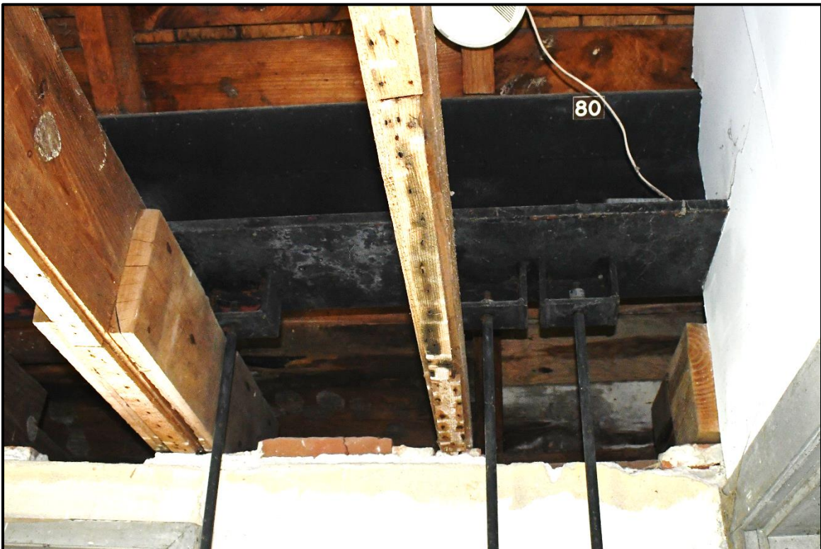
Photo 30: Steel beam located above the main roof attic floor joist located along the north wall of the home.
