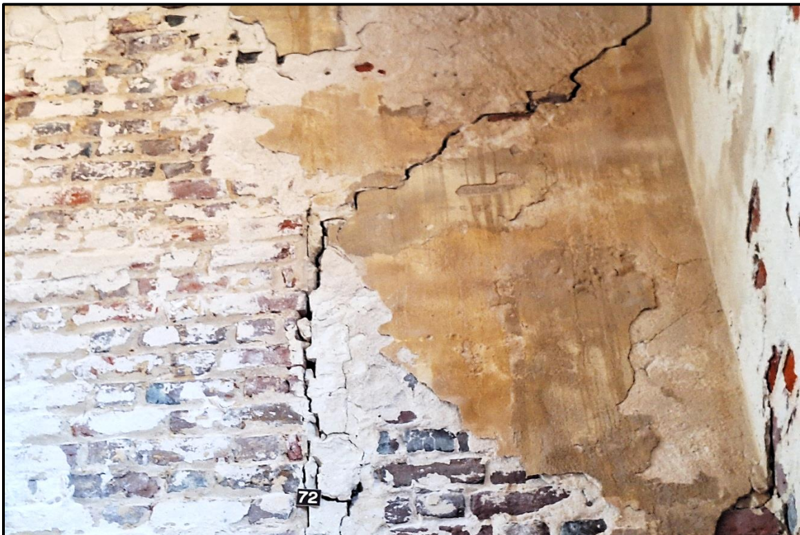
Photo 18: Step crack at the interior surface of the west gable end wall consistent with the location of the exterior crack exhibited in photograph #8 & #9.
