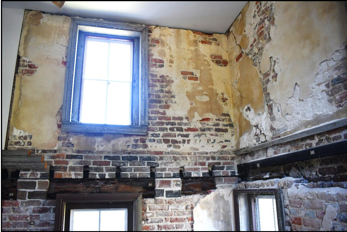
Photo 17: General condition of the existing plaster on the interior walls located at the southwest corner of the home.
