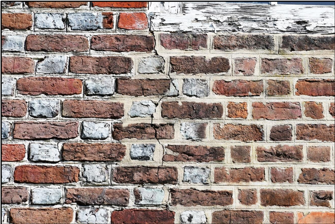
Photo 6: Vertical cracking in masonry observed emanating from the second floor window located above the main entrance along the south elevation.
