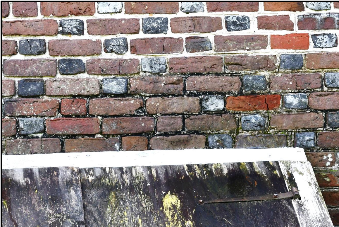
Photo 14: Deteriorated and weathered brick masonry mortar joints located above the cellar door on the north elevation.
