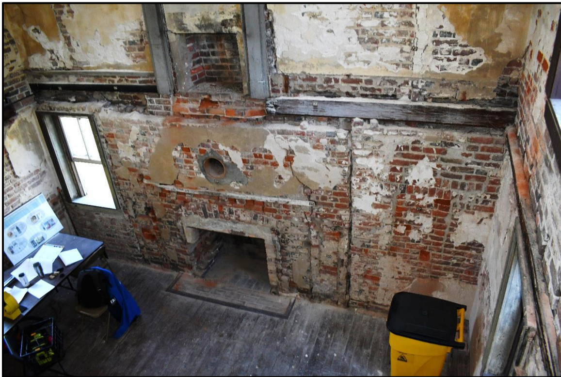
Photo 22: View of the west side of the home showing where the 2 nd floor system had been removed.
