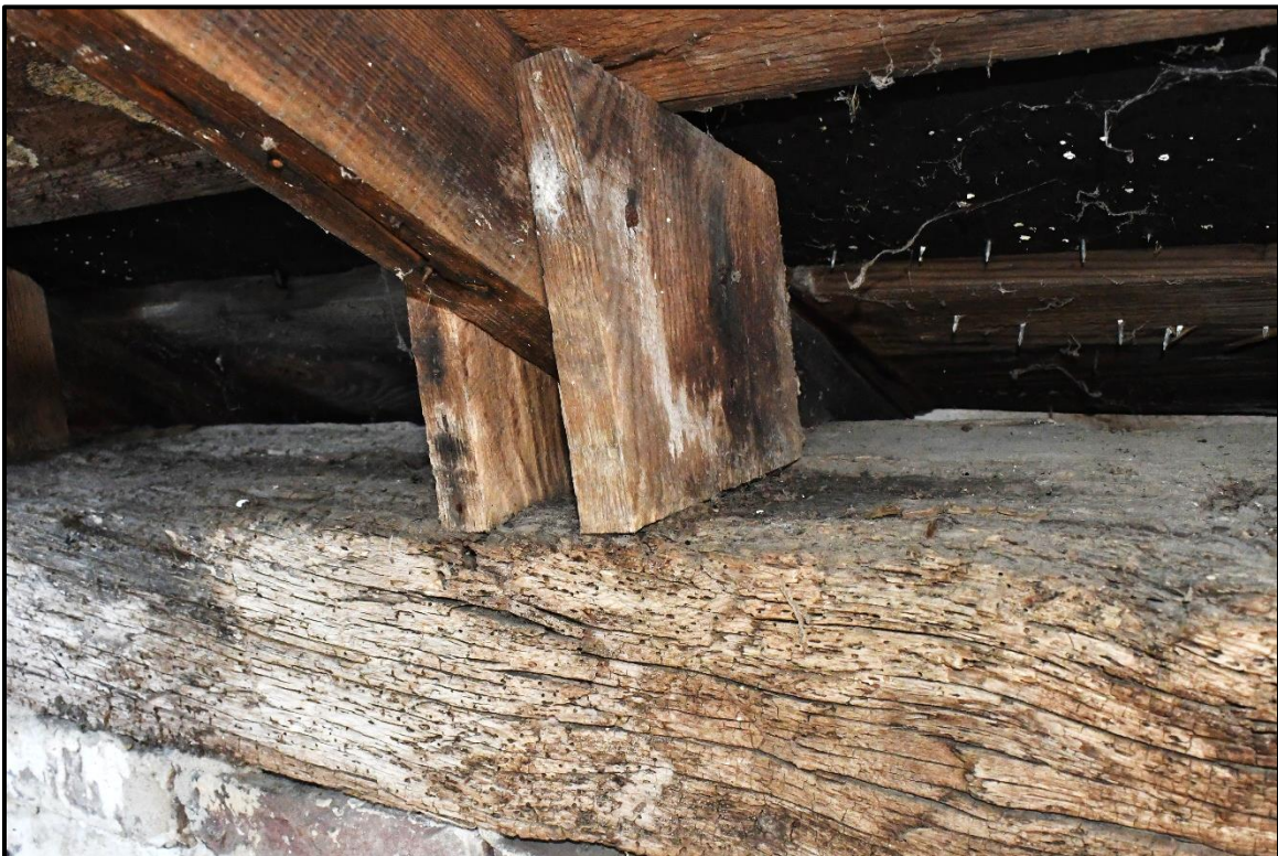
Photo 26: Lower connection of the rear shed roof rafter. Note the deteriorated condition of the timber plate.
