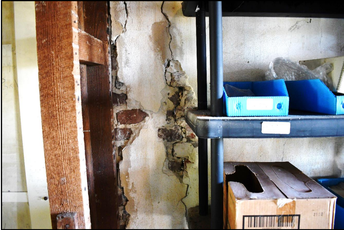
Photo 21: Vertical crack observed in the interior east wall located on the second floor of the entry tower. Note the daylight seen through the crack.
