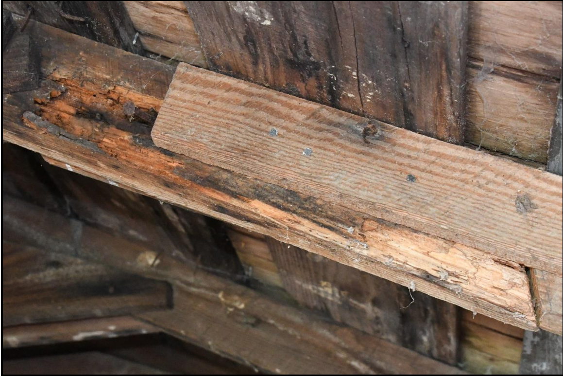
Photo 27: Wood rot or insect damage on a rafter located at the rear shed roof.
