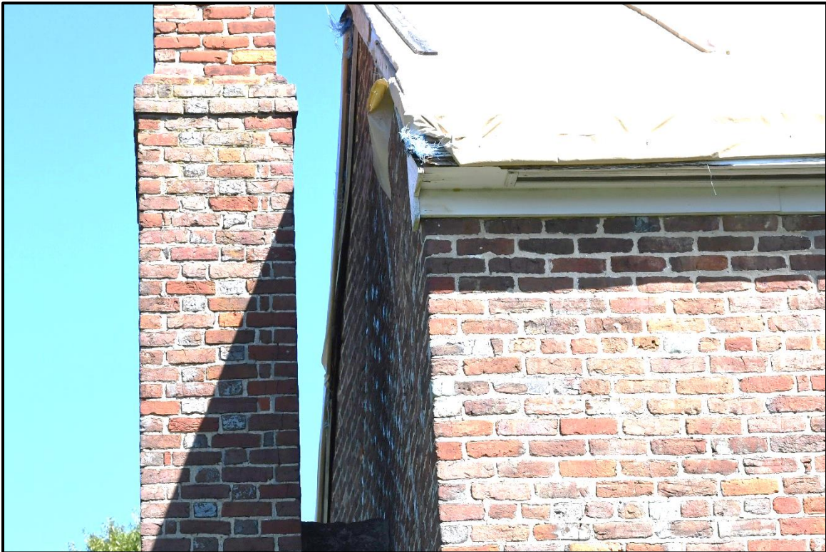
Photo 10: Photograph taken at a view parallel to the west elevation that exhibits the bow in the west elevation gable wall.
