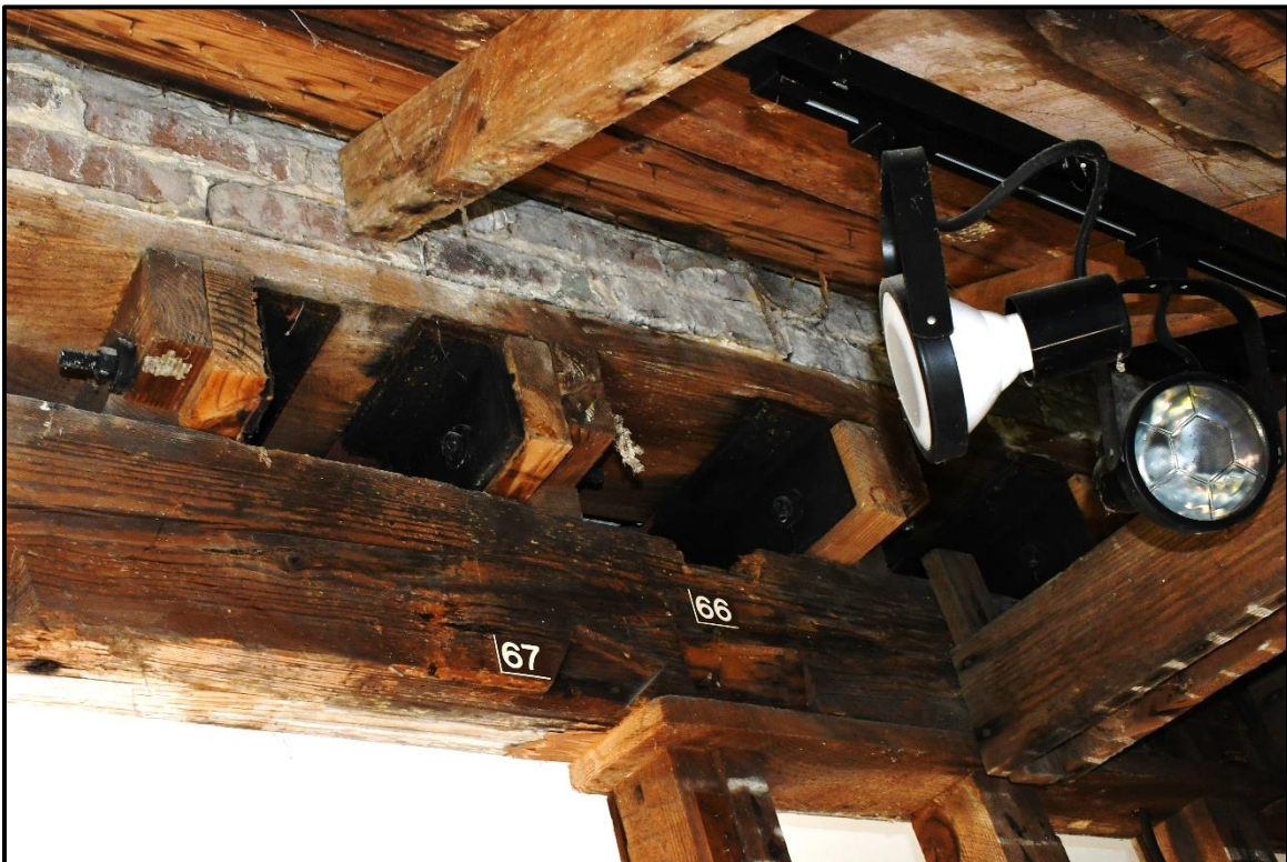
Photo 28: Portion of the second floor system visible from inside the rear shed. Note the supplemental steel angles adjacent to the floor joists.
