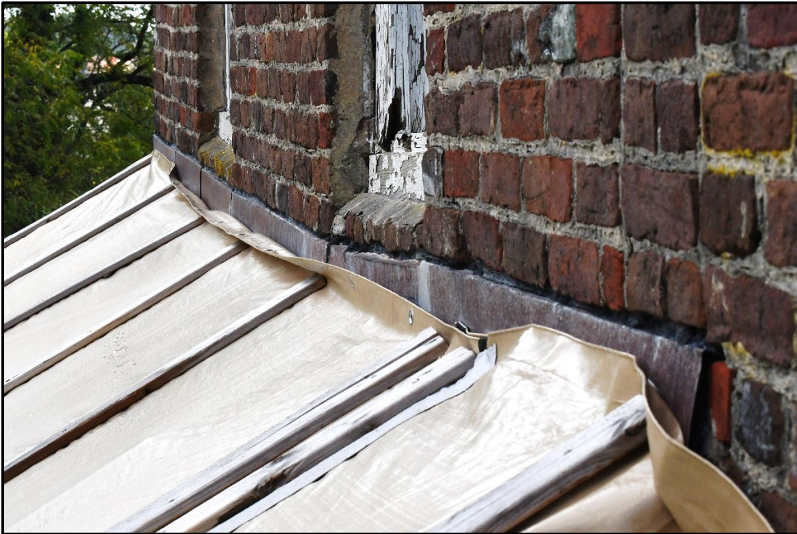
Photo 12: Deflected brick masonry above the shed structure viewed along the north elevation.
