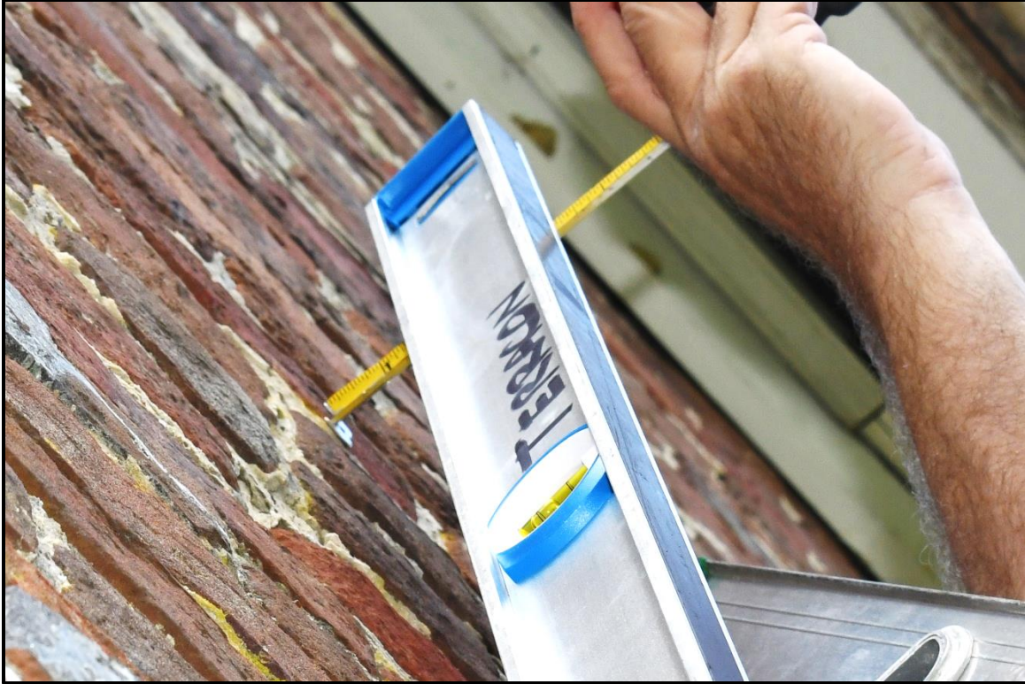
Photo 11: Out of plumb measurement taken at the mid height of the bowed wall area on the north elevation west of the rear shed.
