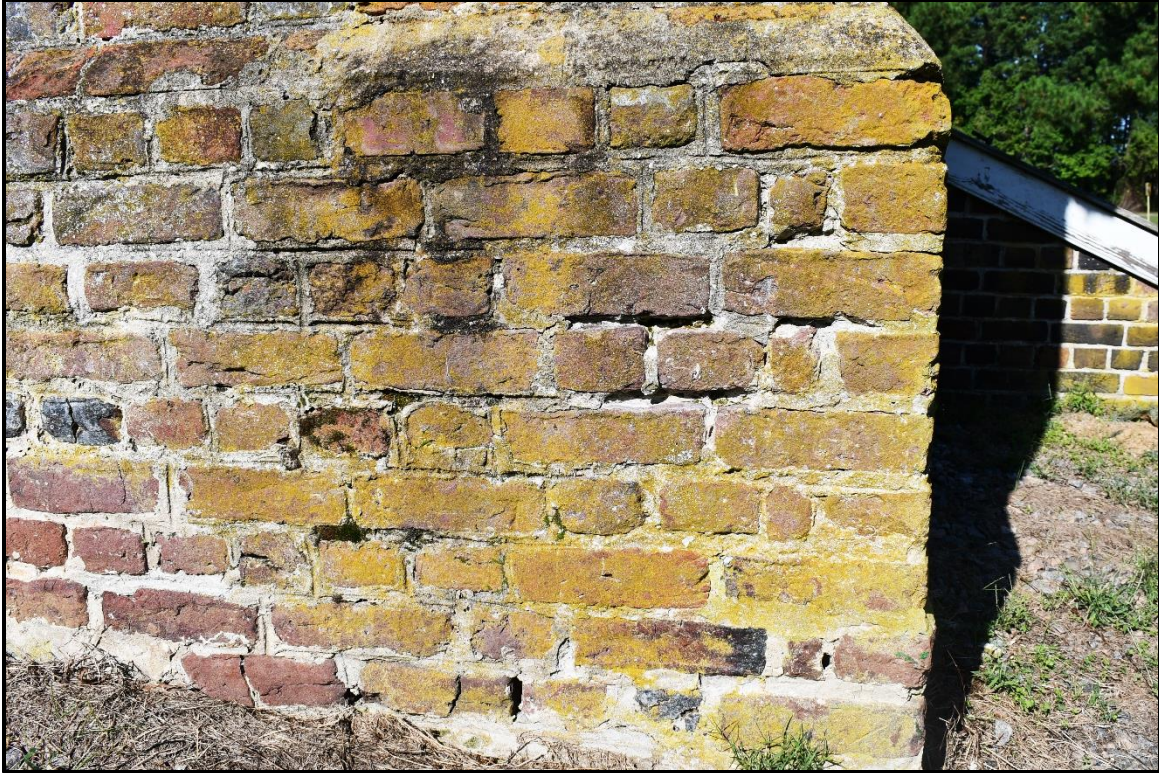
Photo 15: Deteriorated/open brick masonry mortar joints and significant presence of organic growth located at the northeast corner of the building.
