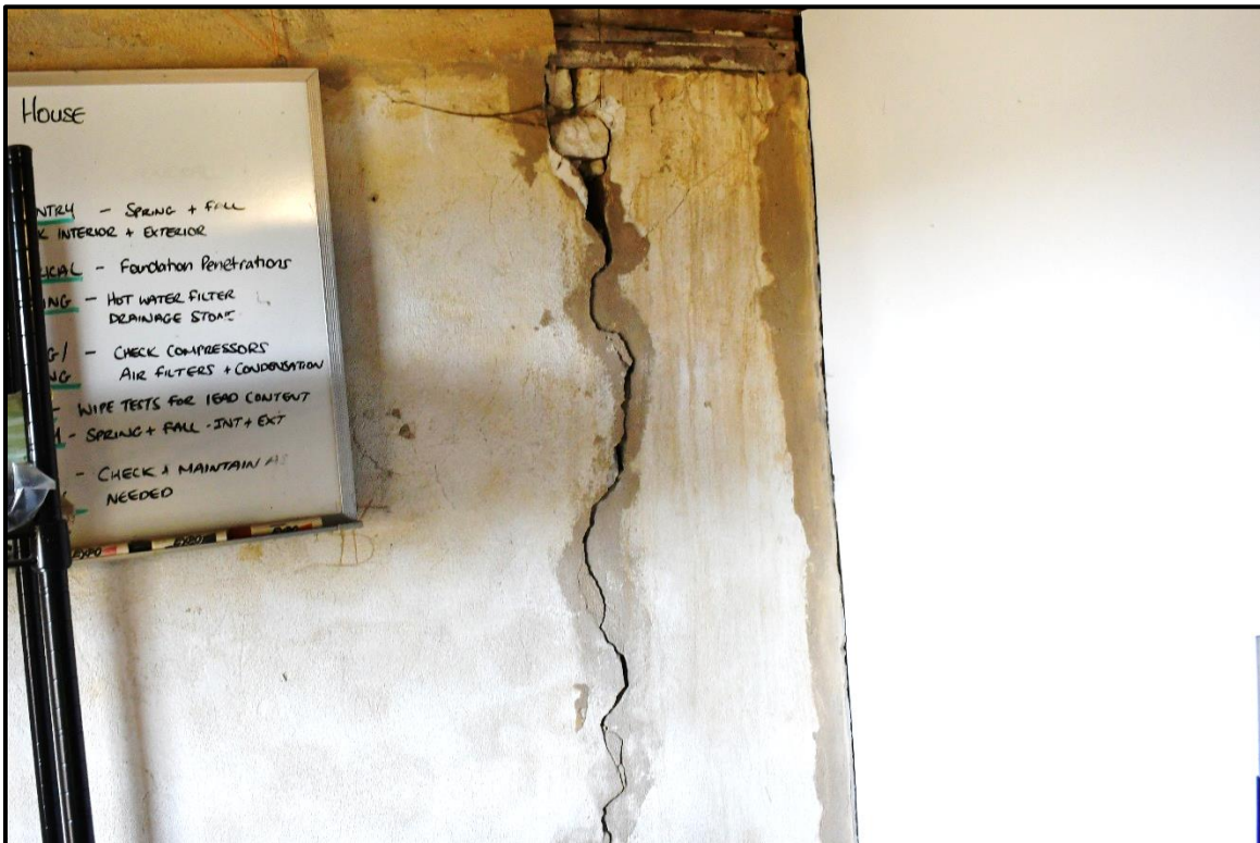
Photo 20: Vertical crack observed in the interior west wall located on the second floor of the main entry tower.
